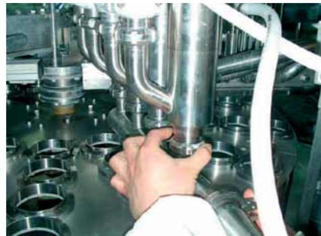
Filling system undergoing upgrade
