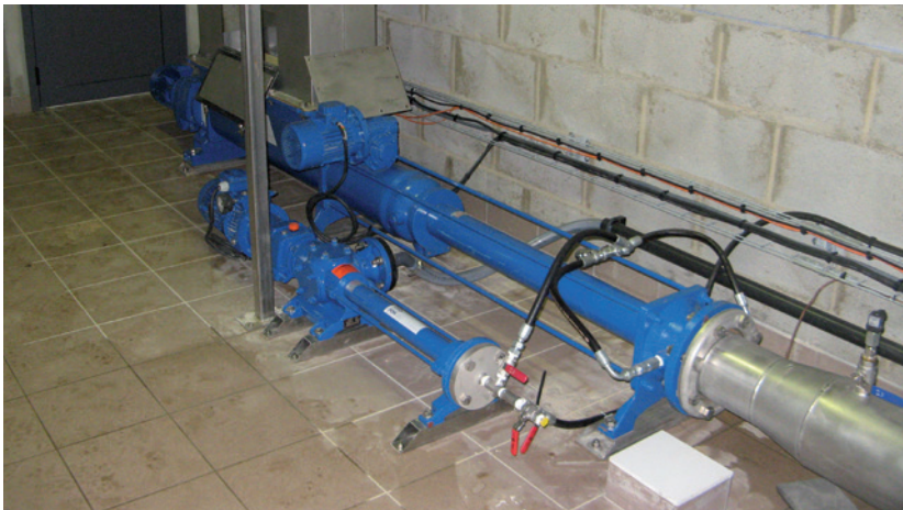
Polymer lubrication incorporated in GBB in transfer of dewatered sludge with or without lime treatment.
