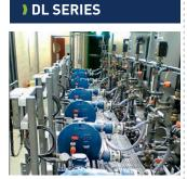
The pump with the reinforced hose for high pressures. Flow-rate: up to 20 m³/h Pressure: up to 15 bar.
