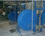
reinforced hose for high pressures. Flow-rate: up to 55 m³/h Pressure: up to 15 bar.
