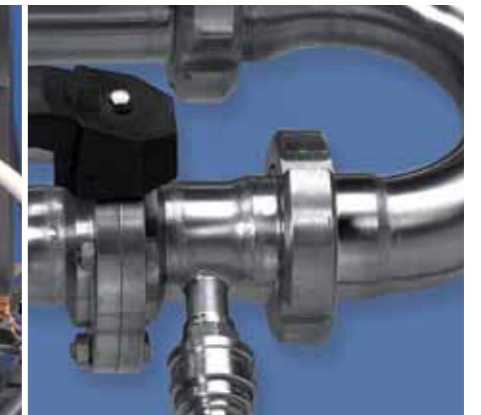
Container suction hose connected to CIP line
