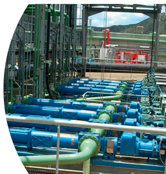
Flocculant pumps with multiple injection points Gold mine, flocculant preparation plant
